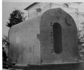
Steel Gothic type Shelter on road side at CIVITAVECCHIA as used in the above position
