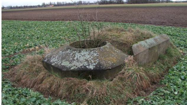
Gothic type Shelter showing additional blast-proof entrance.
